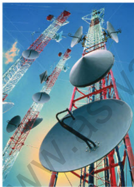
▲ Electromagnetic waves are produced by (and detected as) oscillating electric currents in a wire or similar conducting element. The actual antenna is often much smaller than is commonly imagined—the bowl-shaped structures that we tend to think of as antennas, such as these microwave relay dishes, serve to focus the transmitted beam in a particular direction or concentrate the received signal on the actual detector.
