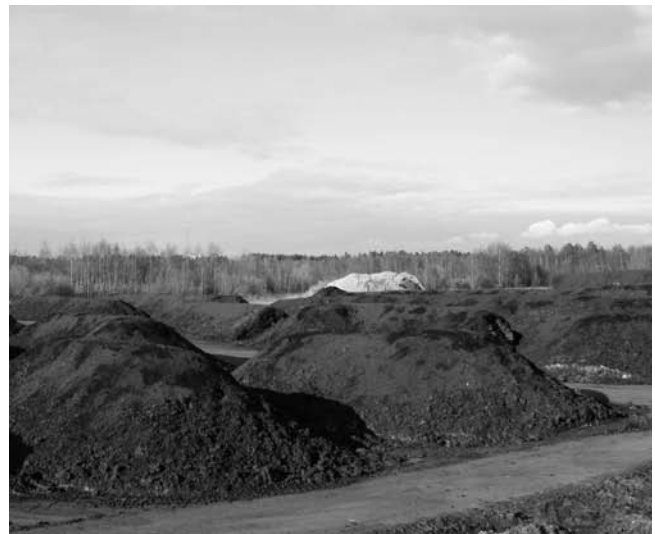
FIGURE 9.9 Soil Biopiles Polluted soil that has been removed from the cleanup site can be stored in piles and bioremediation processes monitored to ensure decontamination of the soil before determining whether the soil can be returned to the environment.
