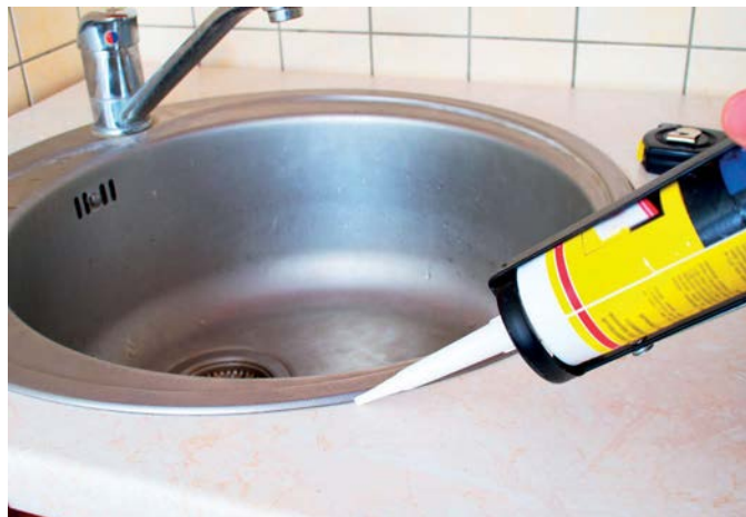
Figure 28.24 Silyl modified polymers (SMPs) are a safer option than traditional adhesives, which use potentially harmful organic solvents.
