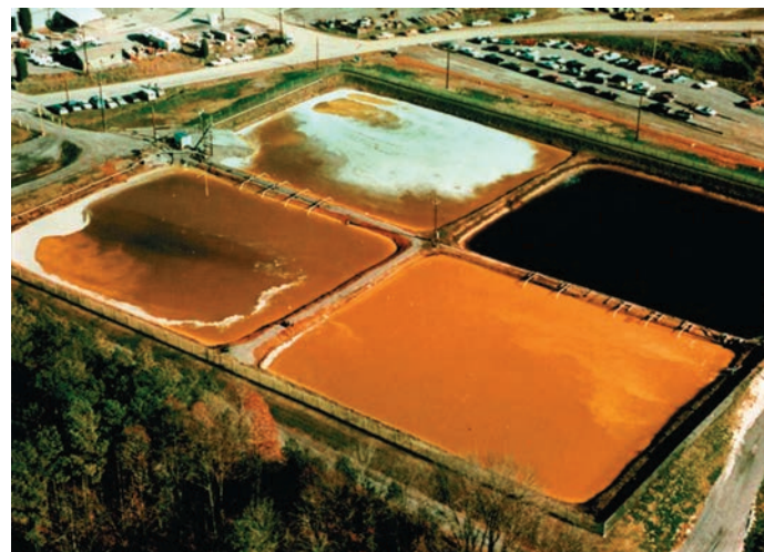
(a) Wastes containing uranium were dumped in these four unlined pits for more than 30 years, contaminating soils and groundwater.
