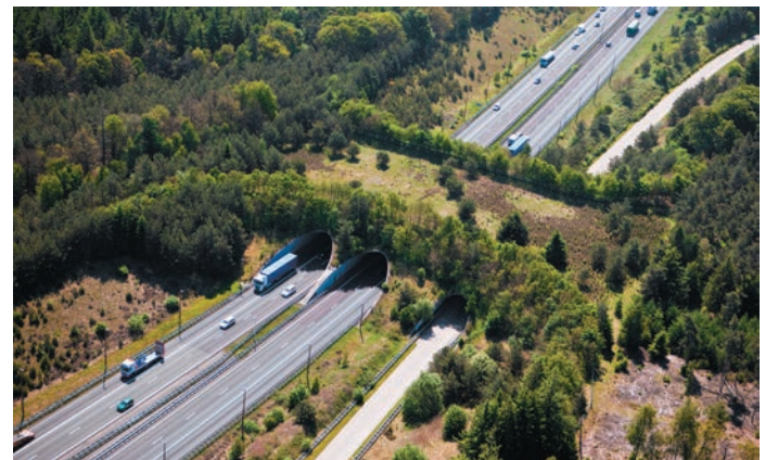
▼ Figure 56.18 An artificial corridor. This highway overpass in the Netherlands helps animals cross a human-created barrier.
