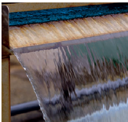
fig. 3.3.6 Ultraviolet light can be used to kill harmful organisms in wastewater.
