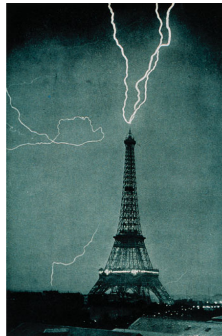
FIGURE 25-25 ■ In this historic 1902 postcard photo, bolts of lightning are shown converging at the top of the Eiffel Tower. The tower is acting as a “lightning rod” protecting people, trees, and other buildings from being struck by lightning.
