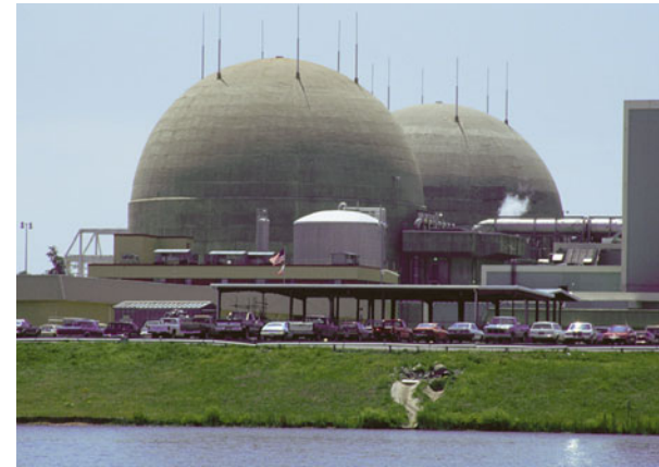
FIGURE 21-11 ■ The North Anna nuclear power plant near Charlottesville, Virginia, which generates electrical energy at the rate of 900 MW. At the same time, by design, it discards energy into the nearby river at the rate of 2100 MW. This plant—and all others like it—throws away more energy than it delivers in useful form. It is a real counterpart to the ideal engine of Fig. 21-7.
