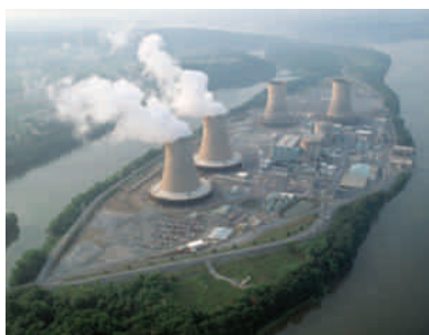
Cooling towers at the nuclear power generating facility on Three Mile Island near Harrisburg, Pennsylvania.
