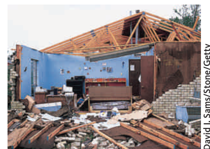
A tornado caused the difference in the air pressures inside and outside this house that tore off the roof.
