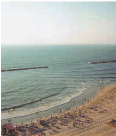
The waves are diffracted as they pass through the openings in the seawall, producing an interesting shape at the beach.
