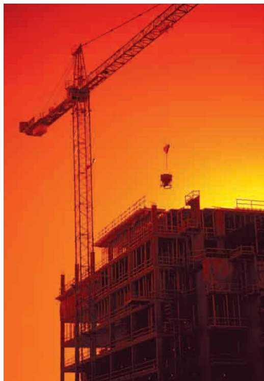
Figure 1.10 Mobile construction cranes can withstand the tension necessary to lift loads of up to 1000 t.
