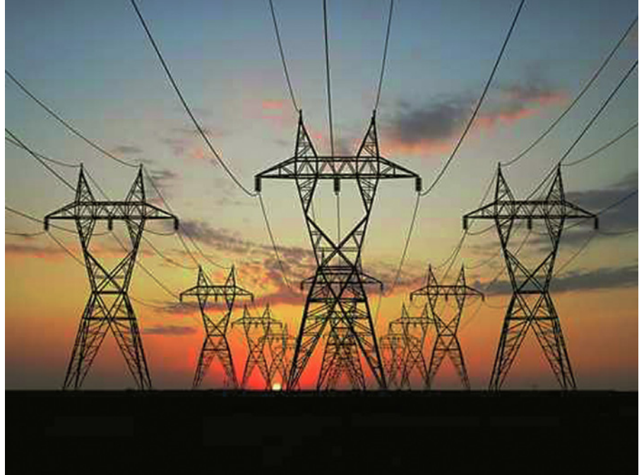
Figure 9.1 Pylons carrying electrical transmission lines.
