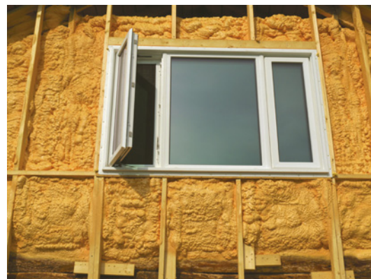
Figure 2.3 Trapped air in this foam makes it an excellent insulator for this house.
