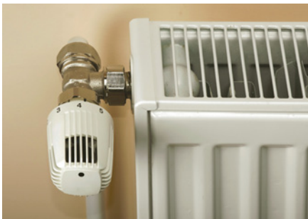
Figure 2.7 This radiator has lots of fins to increase the surface area for heat exchange.
