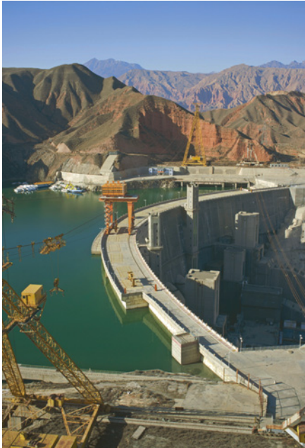
Figure 10.3 This photograph shows the Three Gorges Dam under construction.
