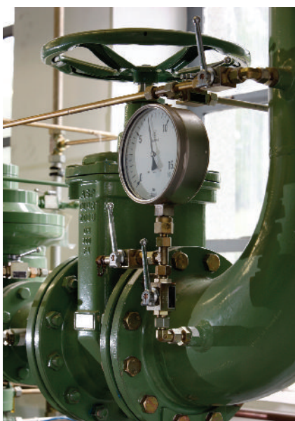
Figure 6.42 A manometer being used
