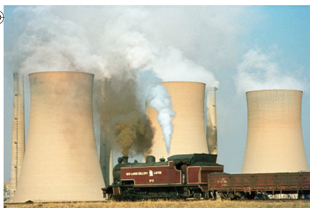
Figure 4.40 An example of a coal-fired power station
