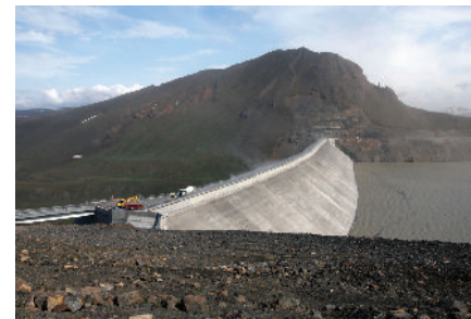
Figure 6.27 Dams have to be thicker at the bottom in order to withstand the greater pressure.
